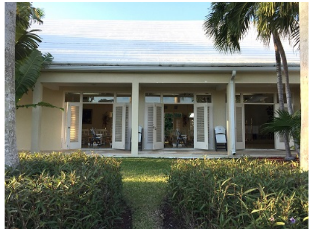
Figure 7. The open southern louvered doors and gallery.
